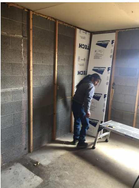
Installing insulation on the Hopi Reservation
