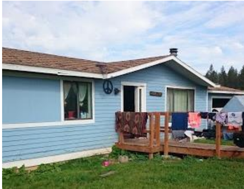
Red Feather starts repairs in July for 4 weeks
